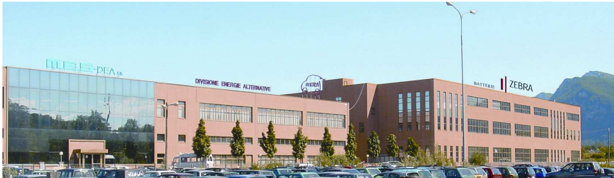
Fig. 11: The New ZEBRA Plant
